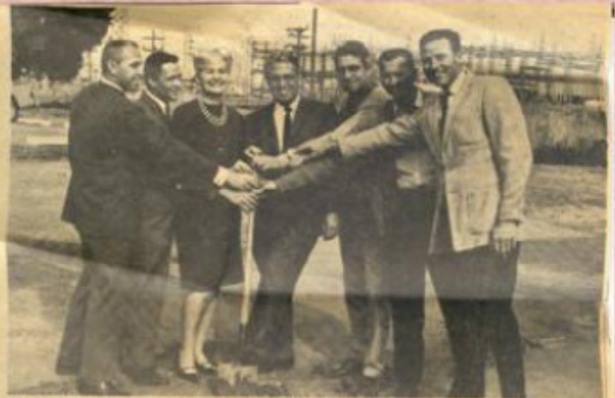
SOD BUSTERS — Mesa Mayor Bert Brown has plenty of helpers as he breaks ground for the new Paris Dance Studio at 345 N. Stapley Dr. From left are Wally Zwingli, vice president of M. J. Hoffman Mortgage Co.; Jack and Ann Paris, owners of the studio; Mayor Brown; Dan Blackburn, contractor; V. L. Shill, planner and architect; and Dr. Fred Lundin, owner of the new dentist building located just south of the construction site. (Tribfoto)
